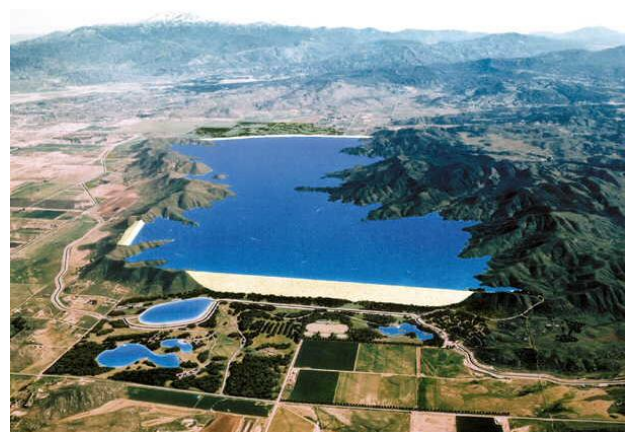
East Dam ( East Side Reservoir)
