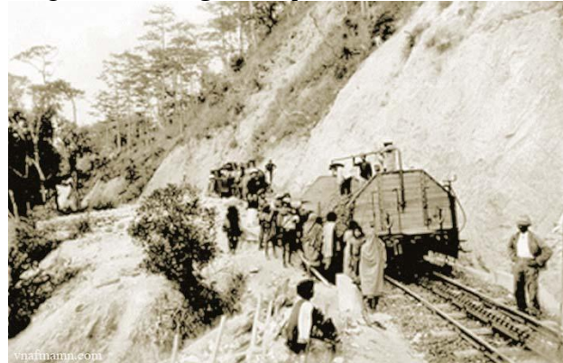
Workers building lay of gravel along the cograil at an unknown section of Song Pha - Dala railroad.
