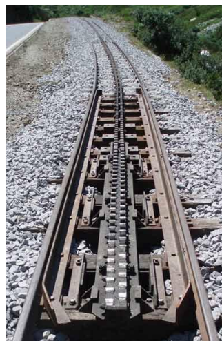
Cog rail of ABT system that has been used on Song Pha - Dalat railway
